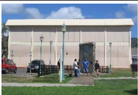
The lowly 1974 air conditioning building is a workhorse, providing cool air to Buildings 6, and 7 (right). The building matches the design of Building 7.
